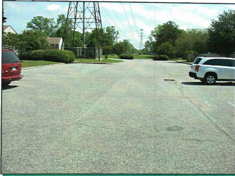
Asphalt pavement overview
