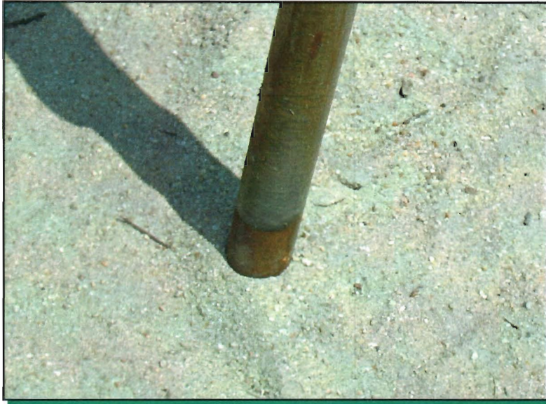
Rusted post of swing set
