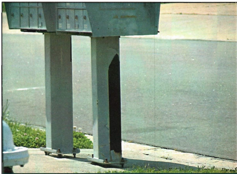
Rusted post of mailbox station (Post Office Responsibility)
