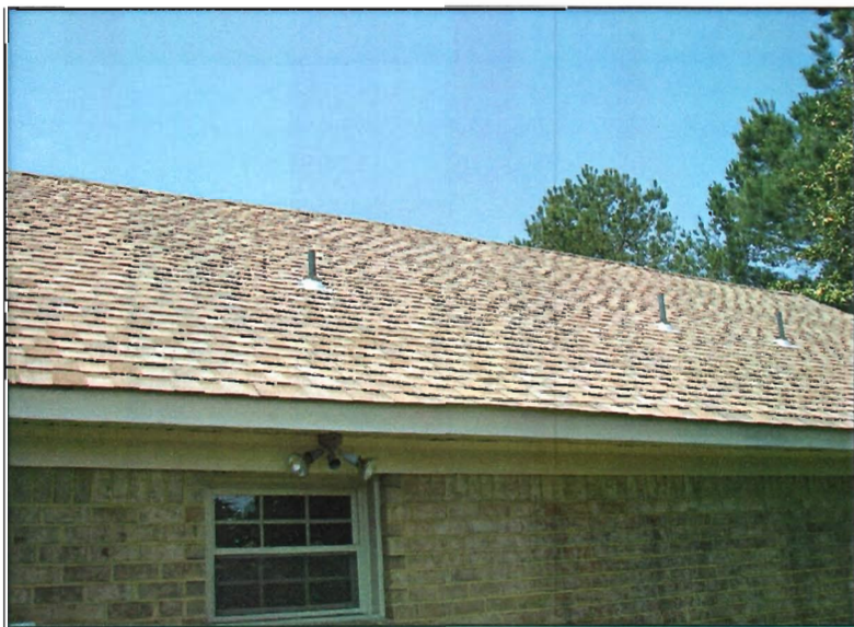
Asphalt shingle roof overview
